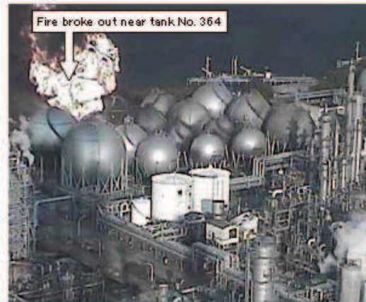
*4. Leaked LPG caught fire.
