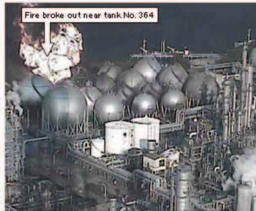
*4. Leaked LPG caught fire.
